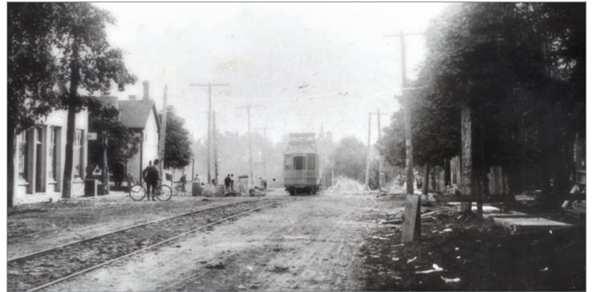
Main Street (Lakeshore) Port Credit, 1906. www.mississauga.ca
