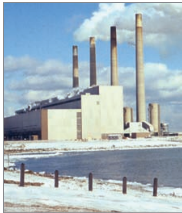
Lakeview Generating Station, 1972. www.mississauga.ca
